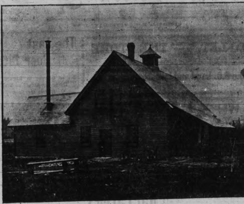
EXTERIOR VIEW OF THE BUILDING. Photo and Half-Tone by B.C. Photo Engraving Co.
